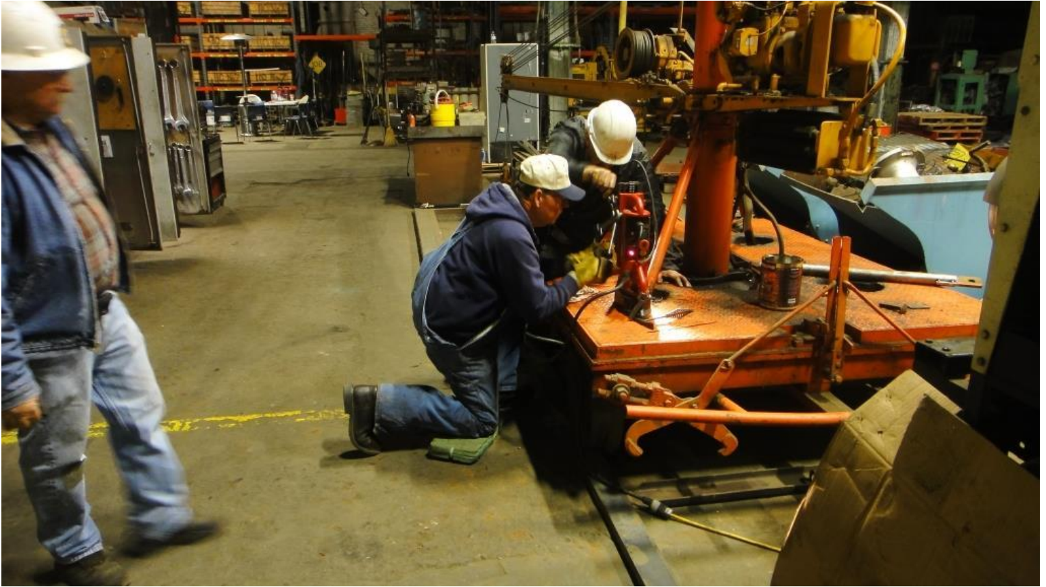
Cliff and Fred engage the magnetic drill-press to open drainage holes on deck of the derrick crane
