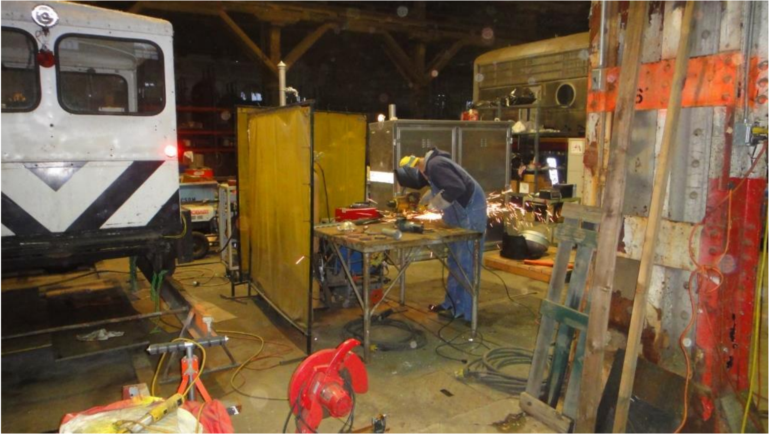
Cliff creates a new support bracket for the derrick crane
